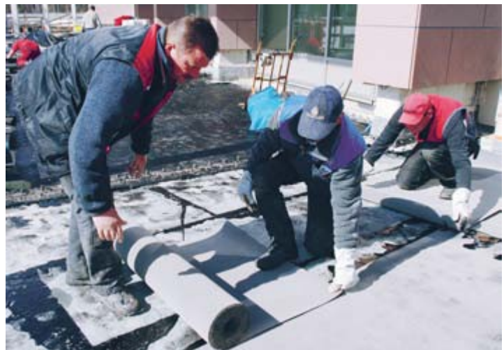
Dacharbeiten am KMCC (Foto: Kaiserslautern American, Airman 1st Class Kelly LeGuillon)
